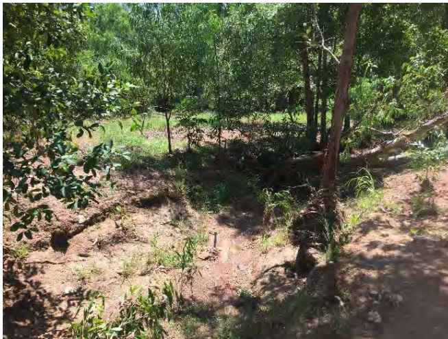
Figure 4-4 Main in sleeve exposed in northern drain
